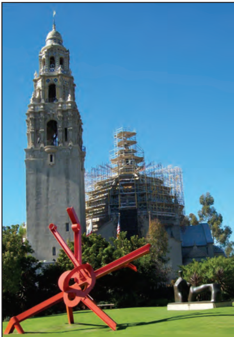
Repairing the Dome. Photo by Curtis Drake.
