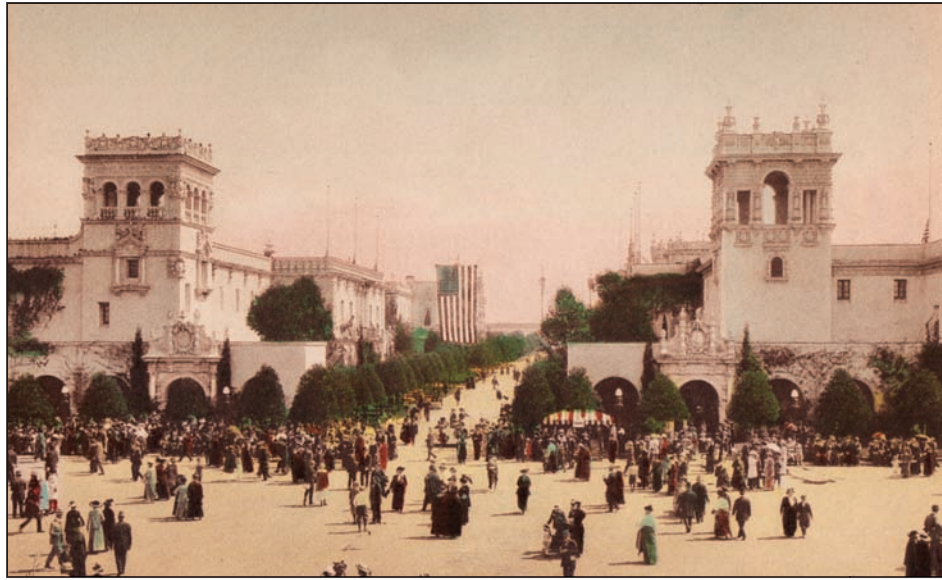
Plaza de Panama, 1915, looking east: Home Economy Building (left) and Foreign Arts Building (now House of Hospitality, right)
