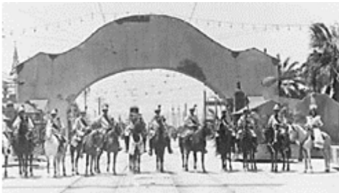
The Grand Marshall and aides at the groundbreaking parade.
