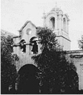
Most exposition buildings, like the Indian Arts Building, were not designed to remain standing after the exposition closed.
