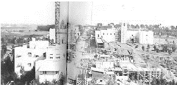
View looking east along El Prado with the framework of the California Building tower beginning to rise.
