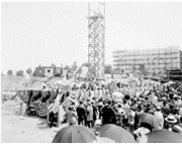
Laying the cornerstone of the California Building.
