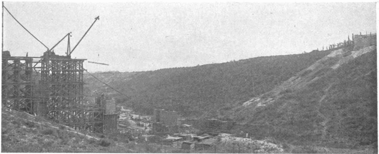
FIG. 4—GENERAL VIEW OF "PUENTE CABRILLA" UNDER CONSTRUCTION AT THE SAN DIEGO EXPOSITION. AT THE EXTREME LEFT IS SHOWN THE GRAVITY TOWER
